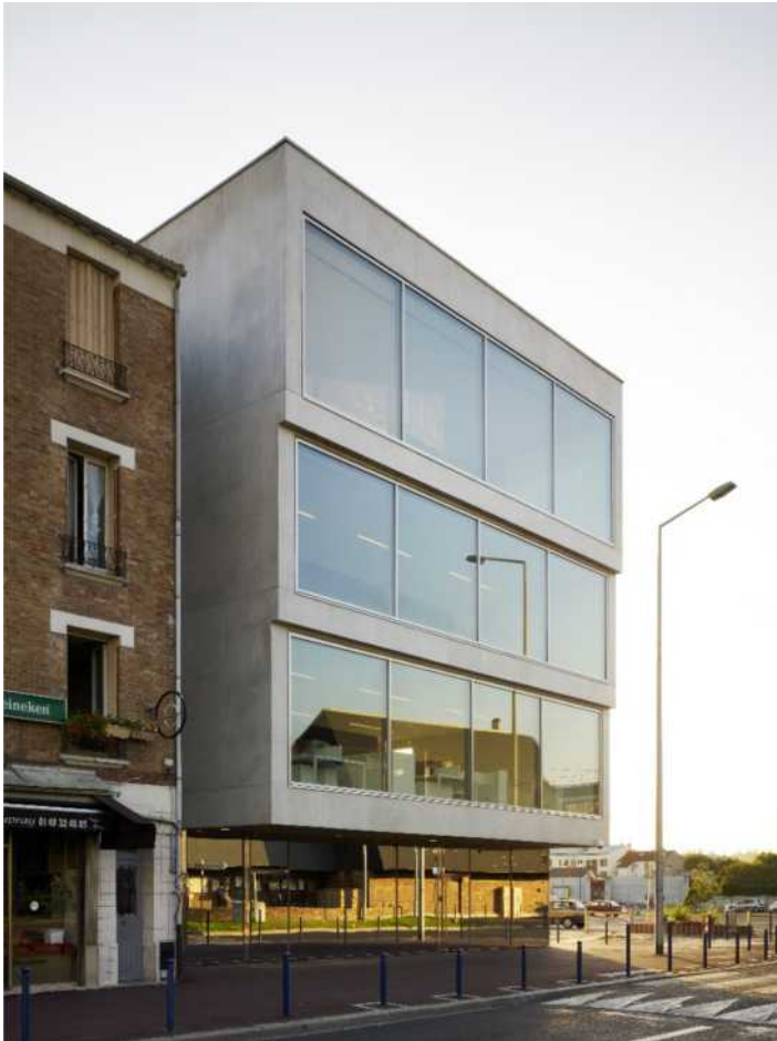
Figure 5. The Drancy Shoah Memorial building, designed by Roger Diener. Photograph © Christian Richters.
