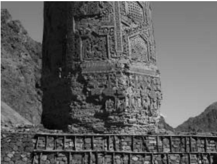
Jam – Gabion protection of the base of the minaret, carried out by UNESCO
