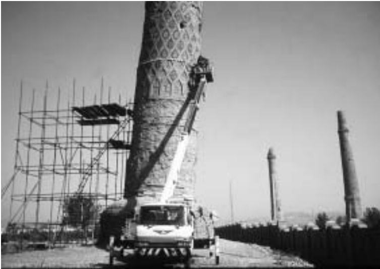
Emergency stabilisation works of the 5th minaret of Herat
